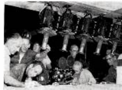
UNIVERSAL demonstrates the working of its new synchronized lighting system. As camera dollies back the lights automatically go on.
